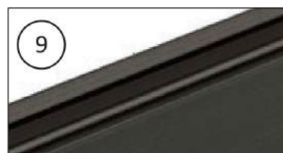
STOREFRONT AND WINDOWS KAWNEER (OR EQUAL) BLACK ANODIZED FINISH
